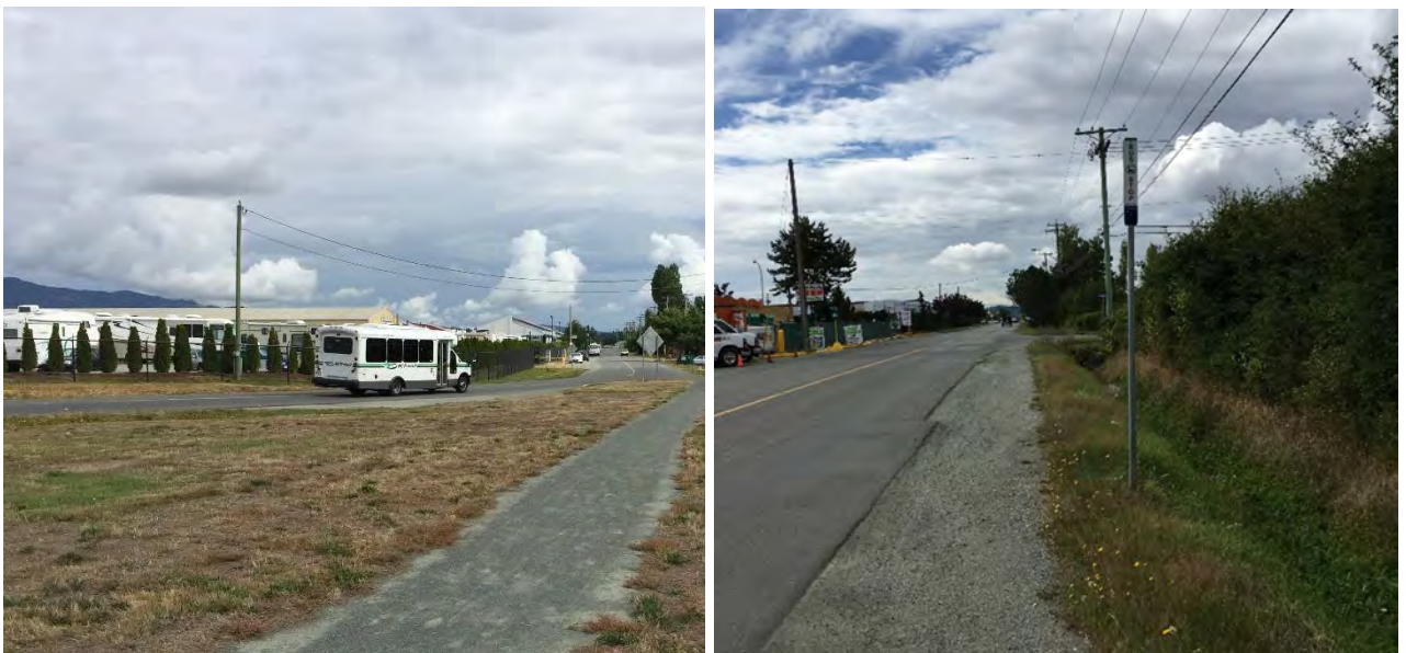
Route 85 (North Saanich) left and shown to the right is example of the bus stops commonly found in the study area, which lack a painted curb, landing bay, and accessible routes to/from the stop.
