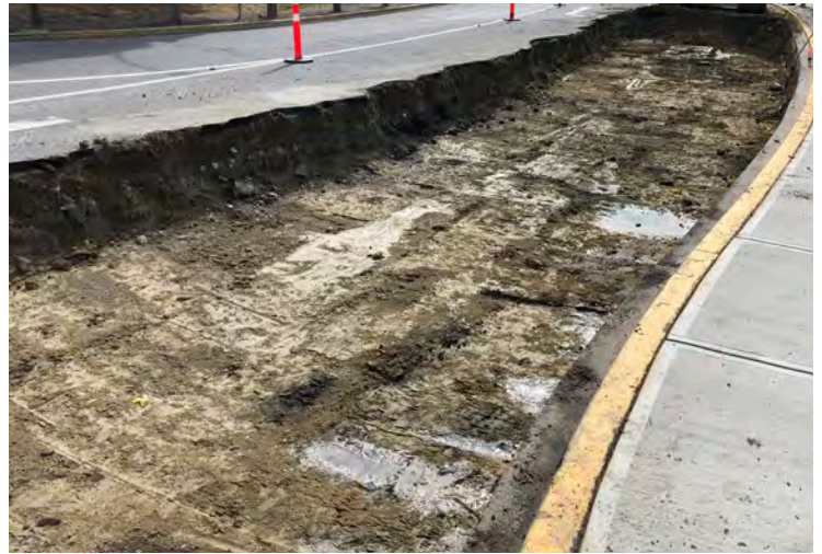
Bevan Avenue Repaving
