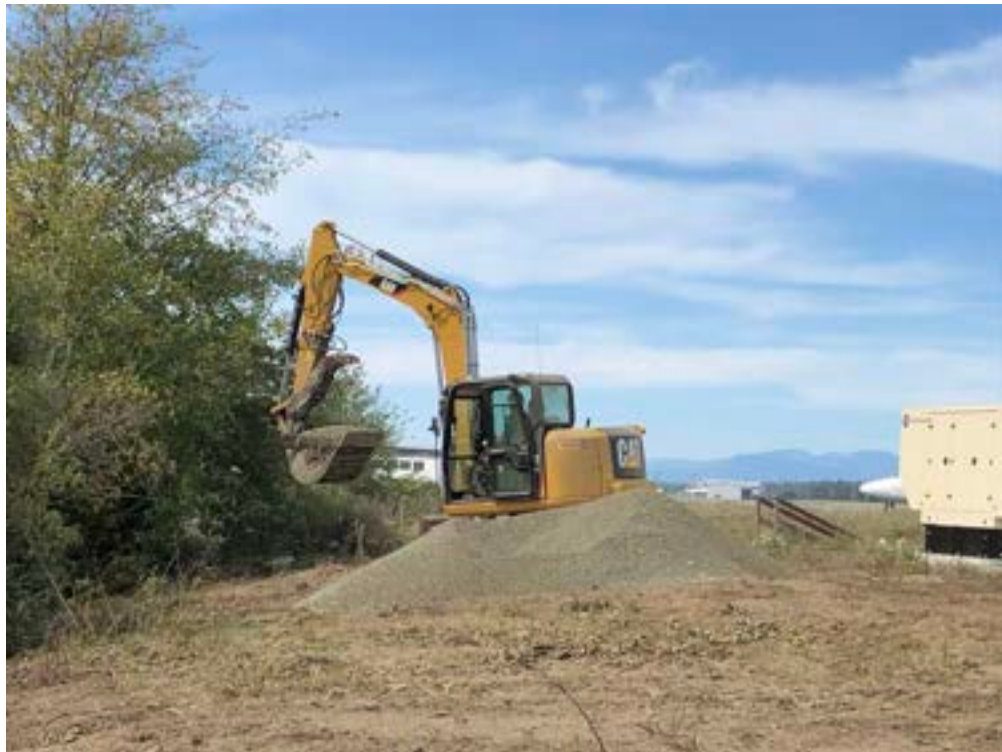
Photo 20: View of Contractor placing Type 1 backfill material in Reach 1A with an excavator.
