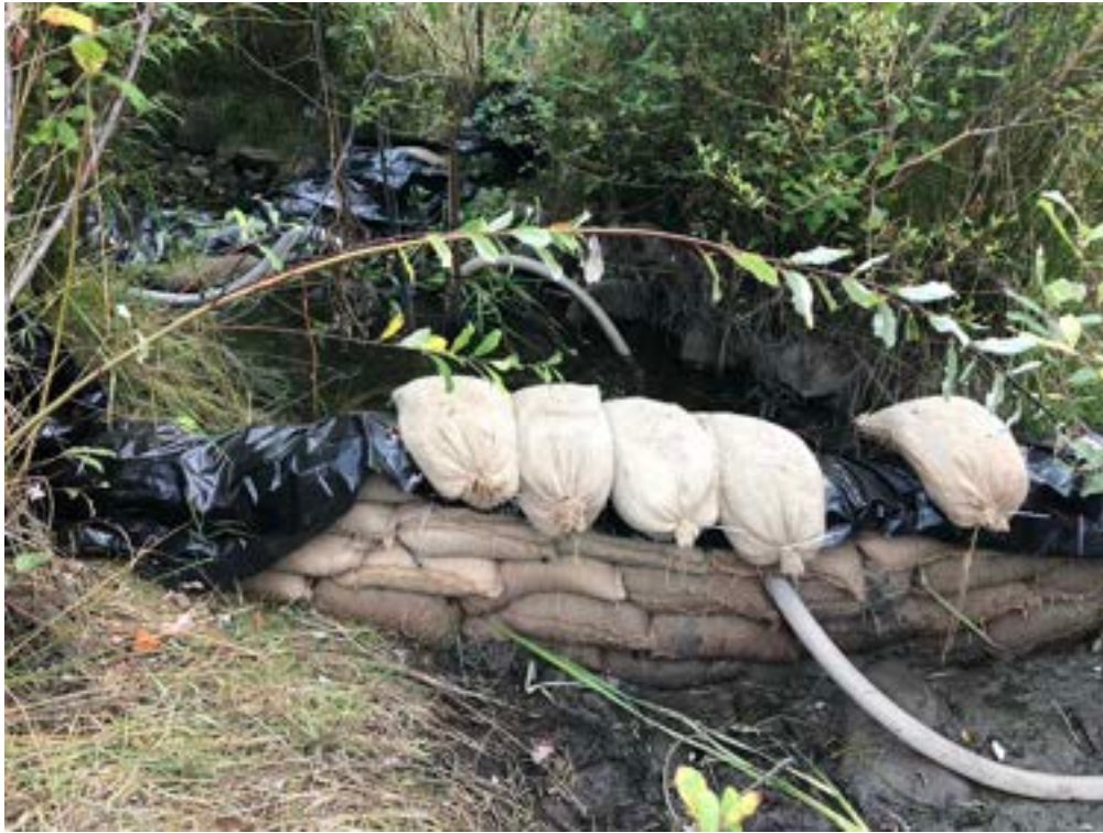
Photo 11: Constructed dam upstream of the remedial extent in Reach 1B.
