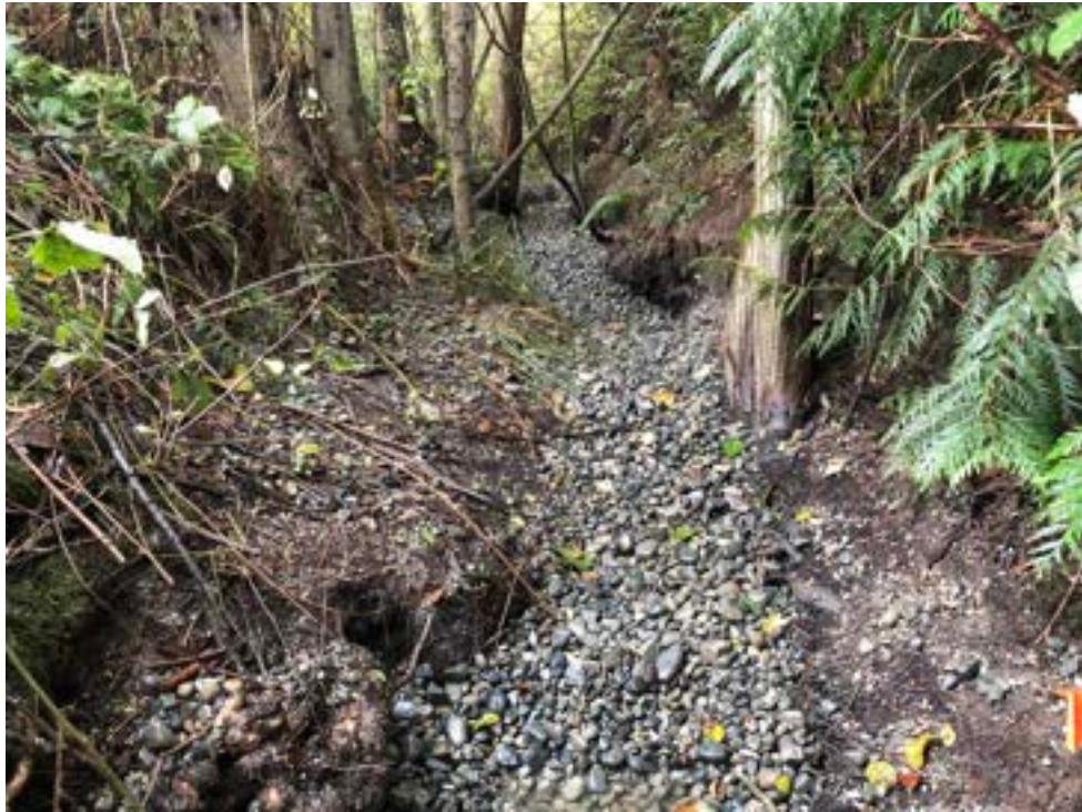
Photo 19: View of backfill (Type 2 blend) shaping and placement in Reach 3.
