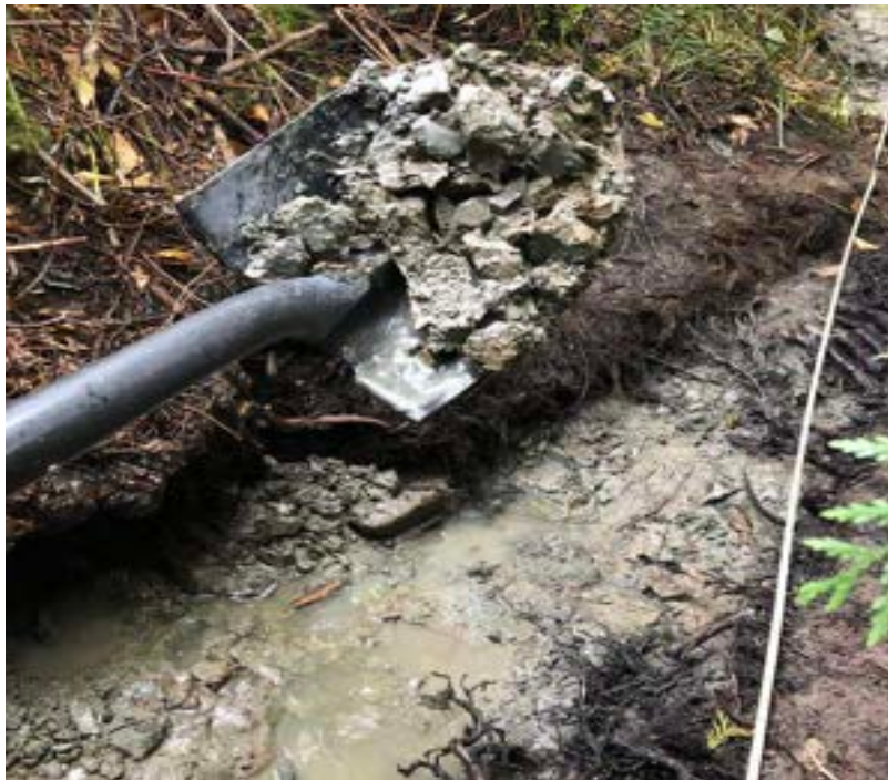
Photo 15: SLR collecting confirmatory samples following hydrovac excavation in Reach 3.
