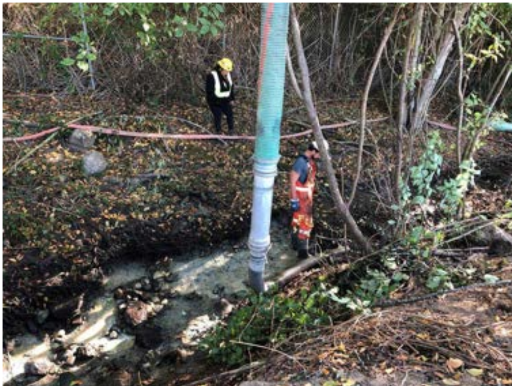
Photo 14: Hydrovac excavation in Reach 1C, Tseycum First Nation archaeological monitor can be seen overseeing the excavation.
