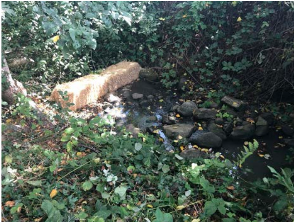
Photo 10: Haybales set up in Reach 1C channel as sedimentation and erosion control.
