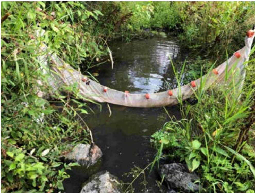
Photo 4: View looking east at the fish stop net installed downstream of Reach 1C excavation limit.
