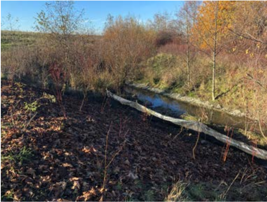
Photo 29: View looking west at an access location along the south side of Reach 1B (west of the large oak tree), riparian planting complete.
