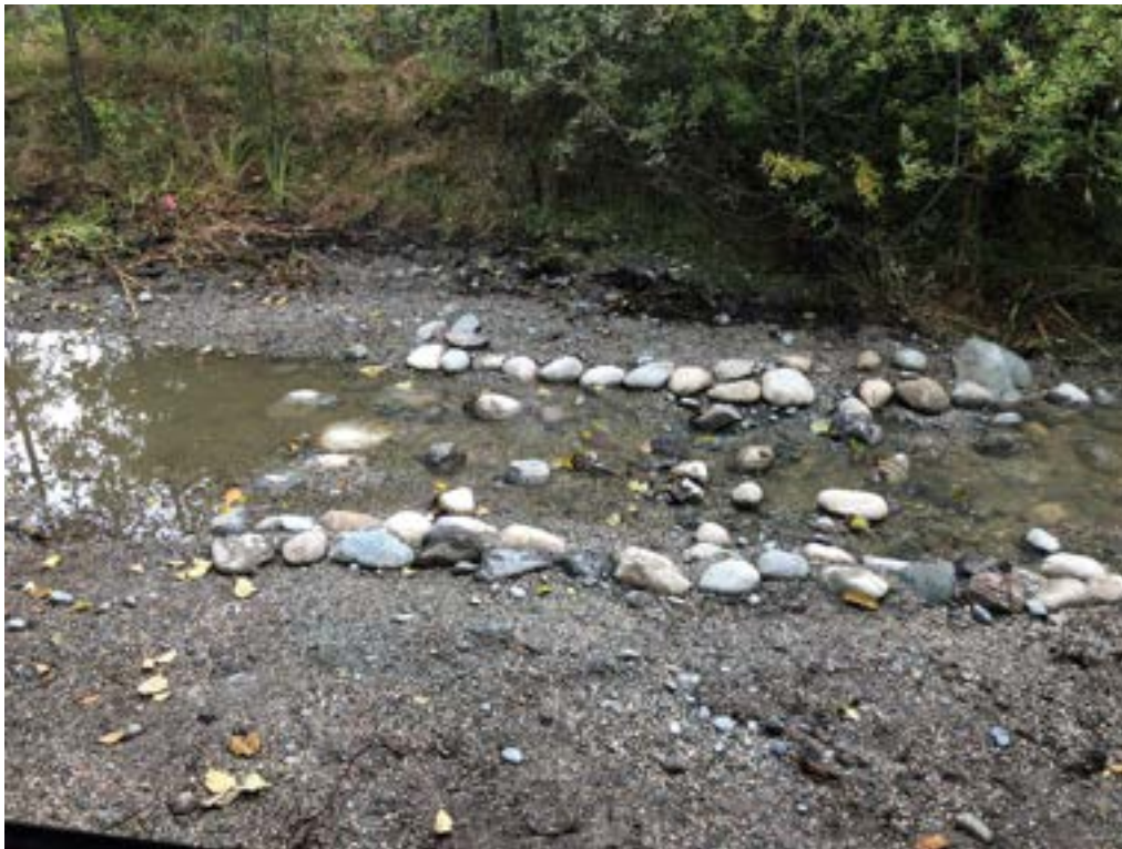
Photo 23: Riffle 3 in Reach 1B after riffle repair and backfill complete.
