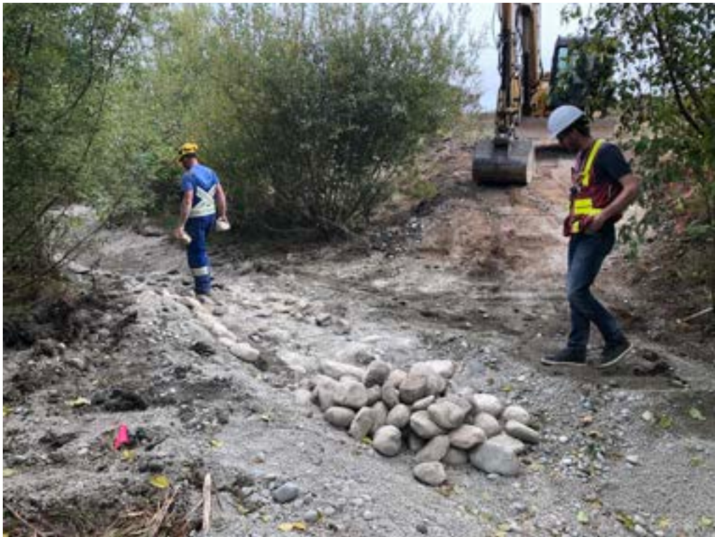
Photo 22: View of KWL personnel inspecting Contractor repairs to riffle 3 within Reach 1B.
