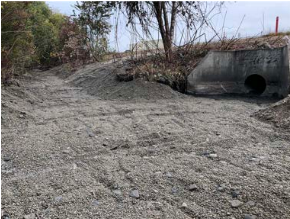
Photo 18: View of backfill (Type 1 blend) shaping and placement in Reach 1A.
