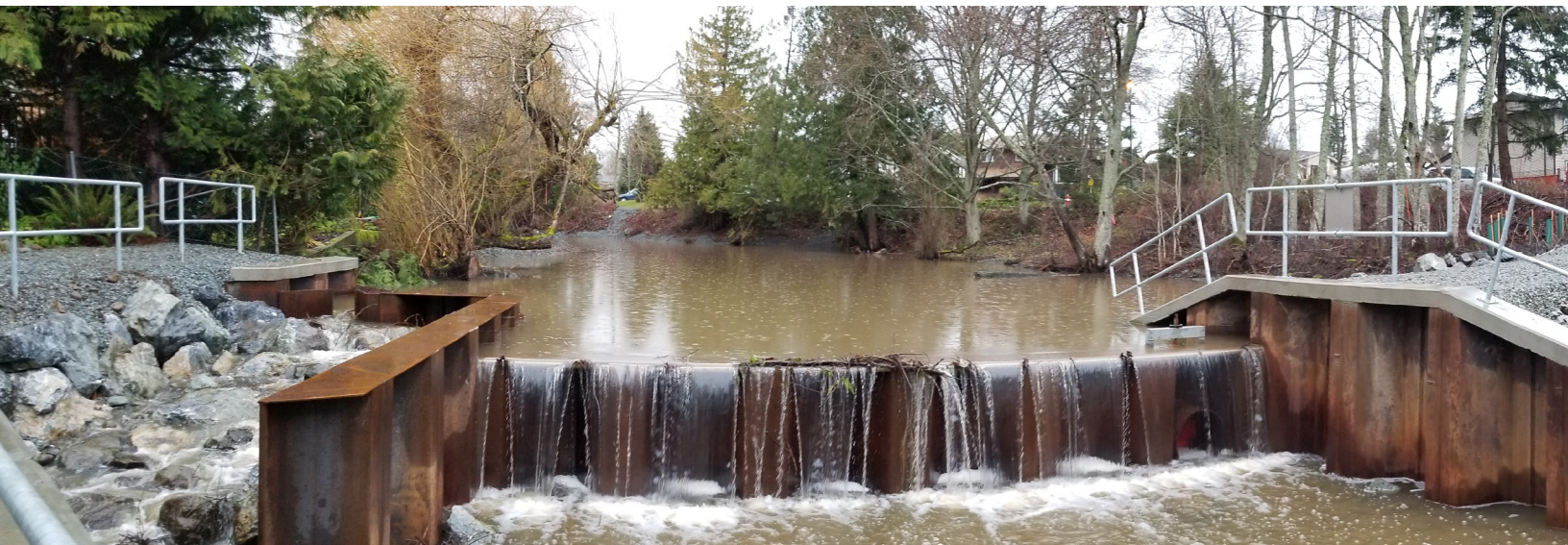
Reay Creek dam renovation
