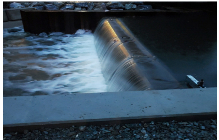
Reay Creek Dam Renovation
