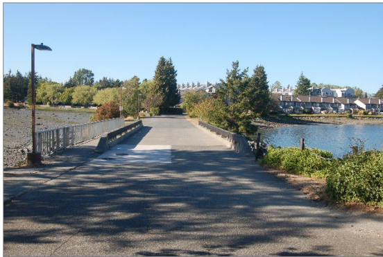
Bridge at Resthaven Island
