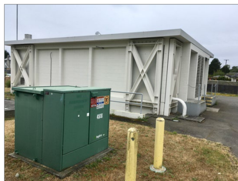
CRD Wastewater Pump Station
