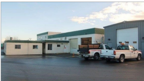
Sidney Public Works Yard
