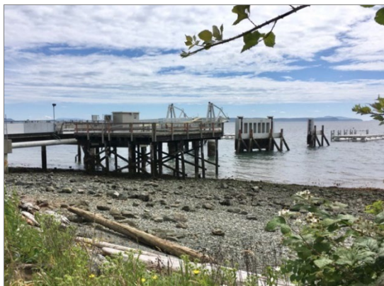
Washington State Ferry Dock
