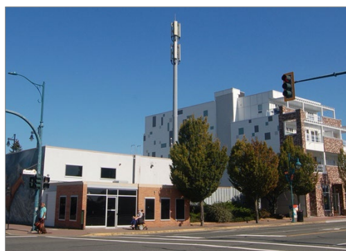
Telecommunications Tower in Sidney
