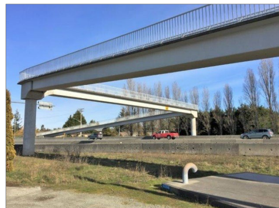
Pedestrian Bridge at McDonald Park Rd
