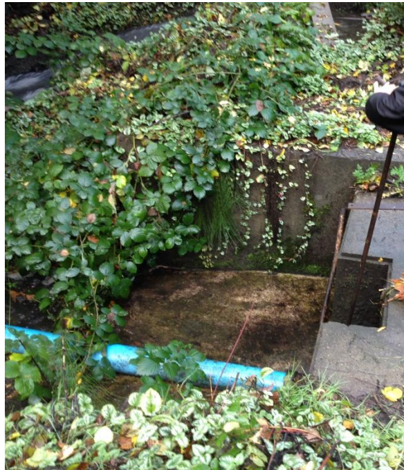
Photo 4: Pond discharge over dam spillway (left & top of right photo) and valve controlled discharge pipe at dam
