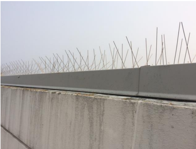
Appendix Figure 22. Spikes in place on the Sidney Hotel and Spa.
