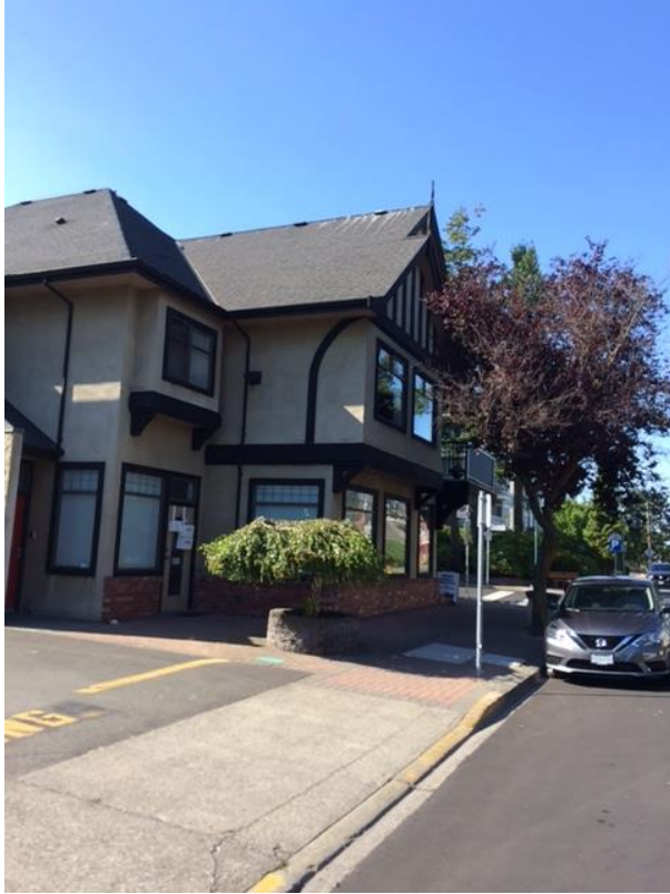
Appendix Figure 17. Another building roof requiring spikes.
