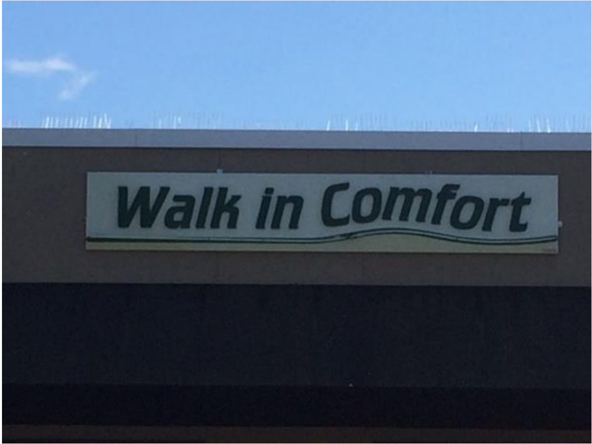
Appendix Figure 12. Spikes in place on a low commercial roof.
