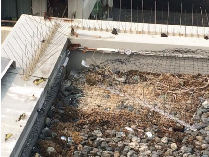
Appendix Figure 33. A typical gull nesting attempt thwarted by the use of netting.
