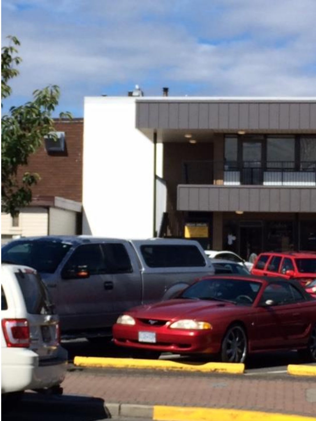
Appendix Figure 4. It is also important to install gull deterrents on smaller infrastructures like ventilator shafts; otherwise despite spikes on the peaks and edges, the gulls will use them.
