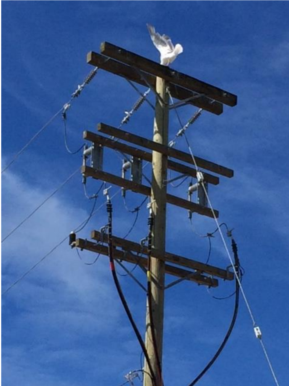
Appendix Figure 3. A close-up of a hydro pole with a gull using it. Exclusionary devices may need to be installed on all of the cross arms.
