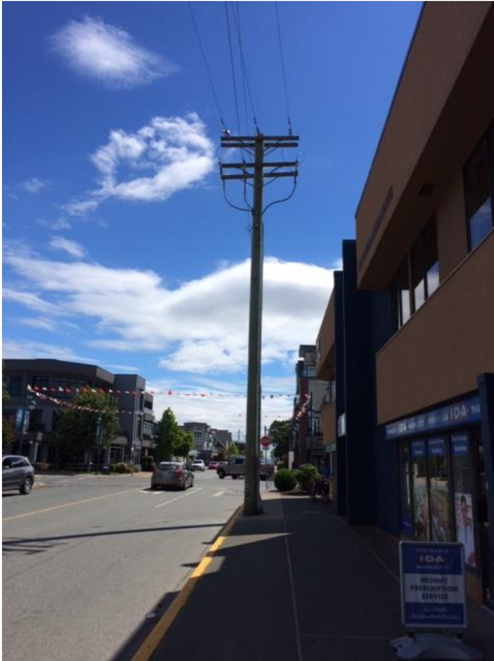
Appendix Figure 9. Another favoured hydro pole on Bevan Ave.
