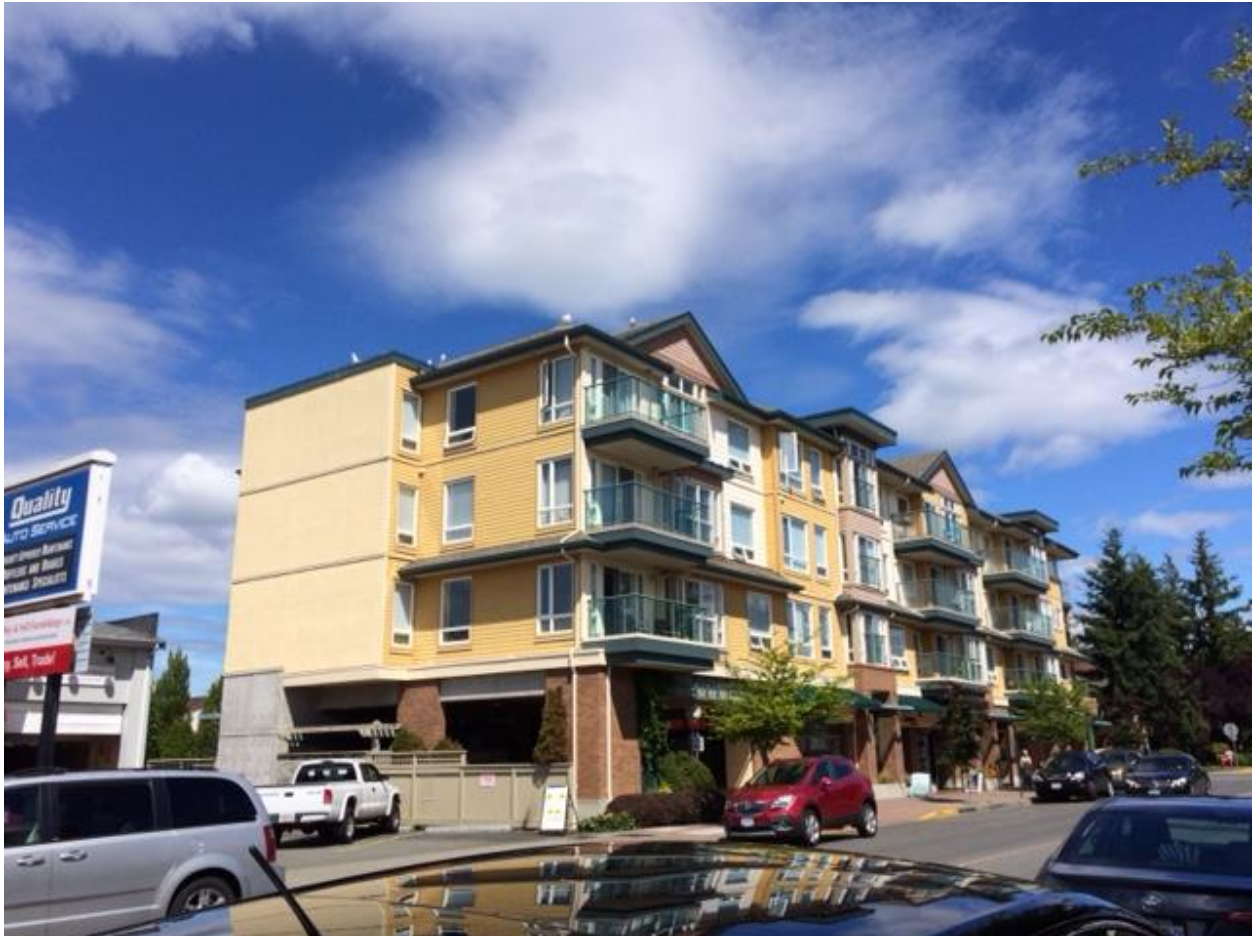
Appendix Figure 6. On that favourite 'gull' building with no deterrents, the birds prefer roosting on the edges and on the peaks to allow for good observation of potential food sources and of predators.
