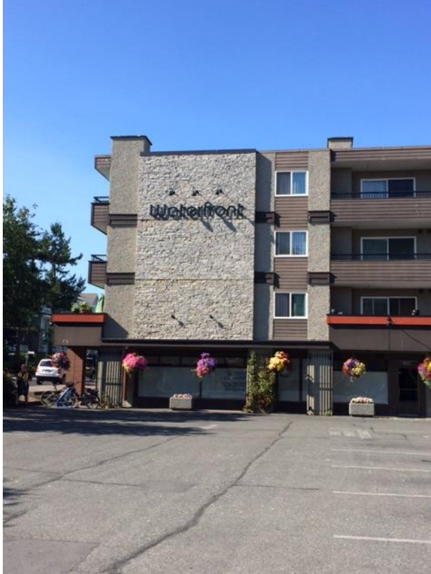
Appendix Figure 15. This building needs gull deterrents.
