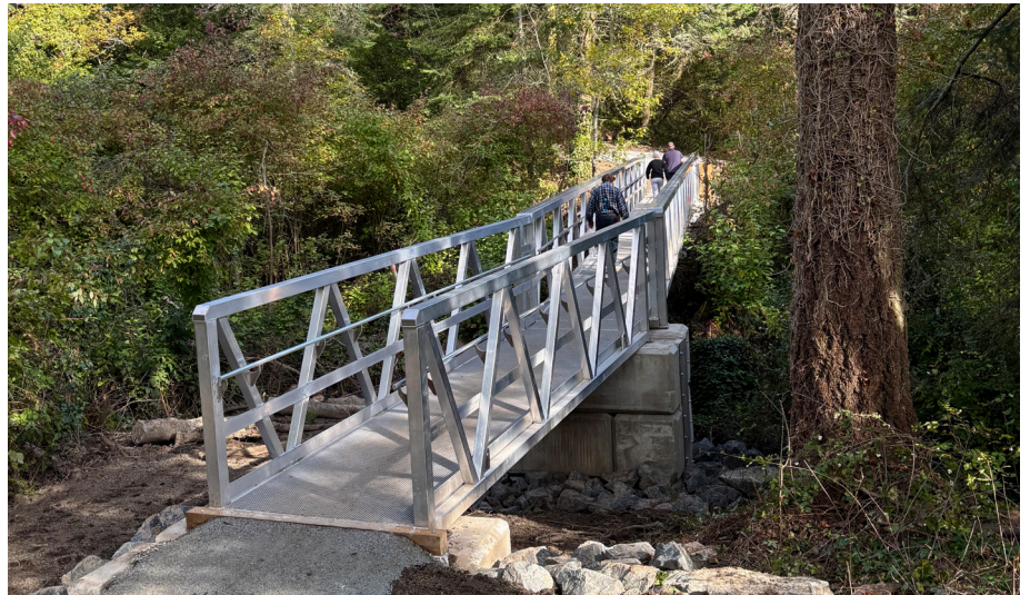
||| A new pedestrian bridge over Reay Creek opened in October.
